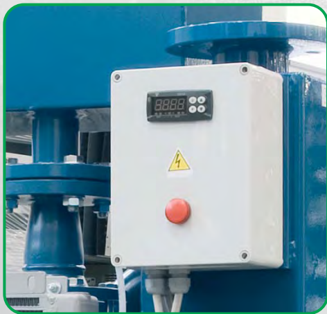
Electronic heat regulator for detection and oil temperature alarm
